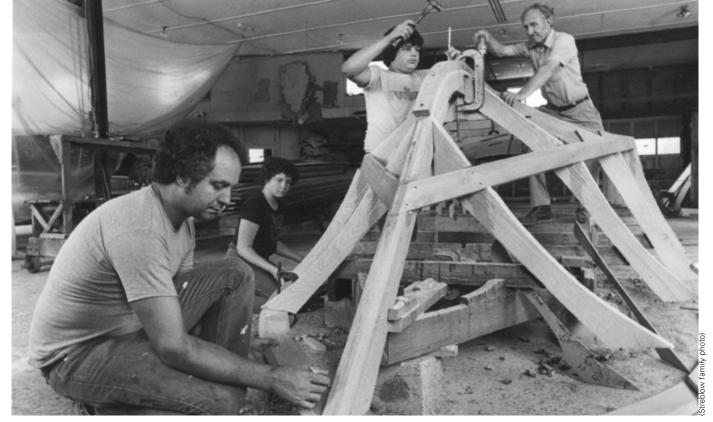
It's all in the family, as three generations of Streblows work together on a boat. Kneeling in front, current owner Randy marks alignment, while daughter Kris, also kneeling, helps to hold the board steady. In the meantime, Randy, Jr., taps a bolt into the hole just drilled by Grandfather Larry, far right.
