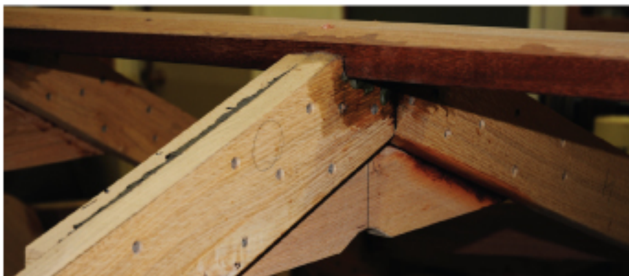
BELOW: Joints are sealed and bedded in fungicidal mastic.
